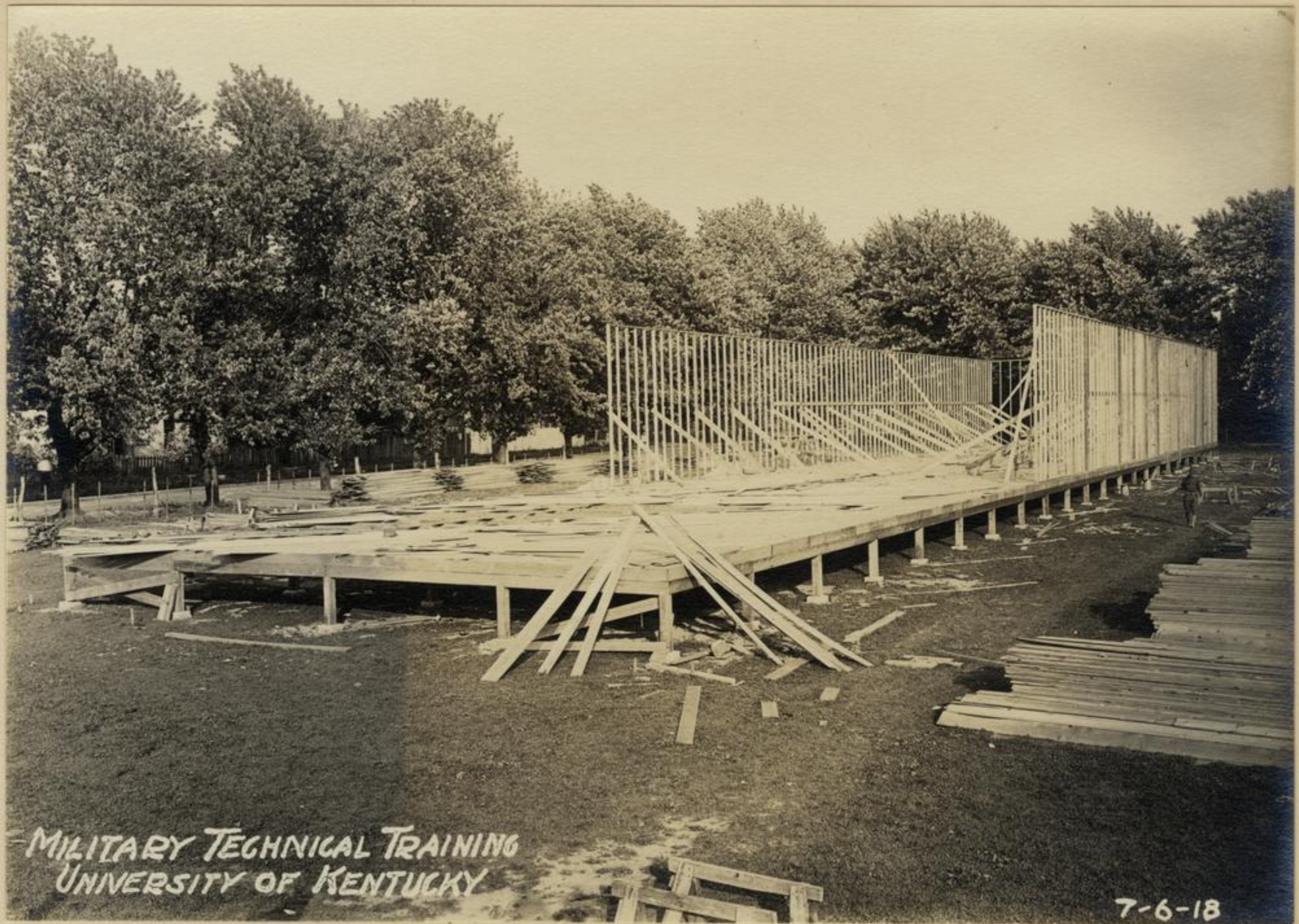
Construction of Barracks by Soldier Mechanics on the Campus University of Kentucky, Lexington, Kentucky
