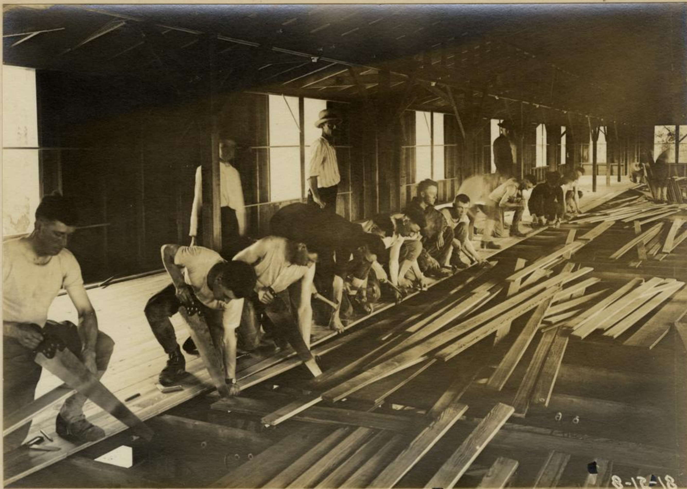
Carpenters Laying Floor in New Barracks
