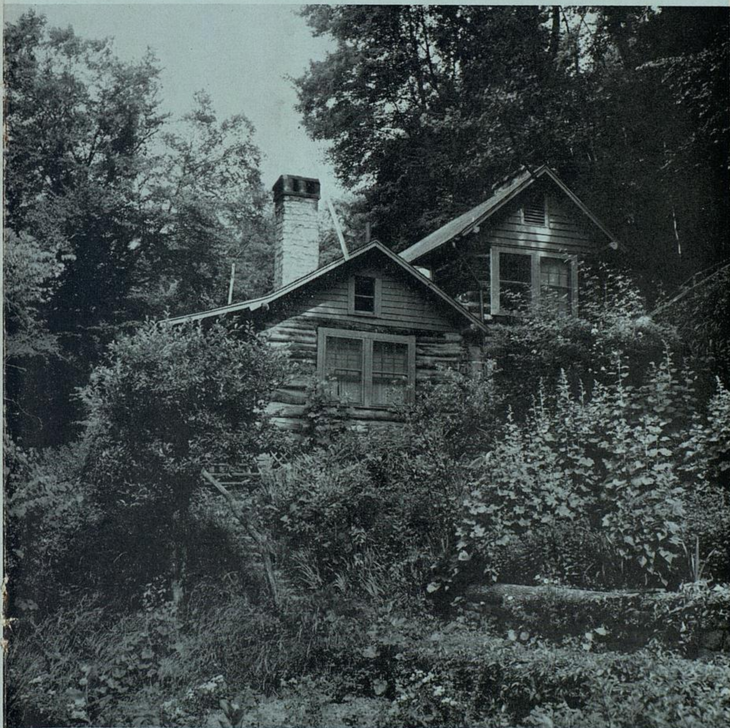
Lower and Upper Cabins and "Blossom Patch" at Wendover
